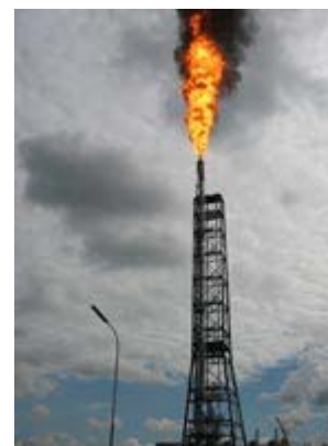
Flare in operation.
